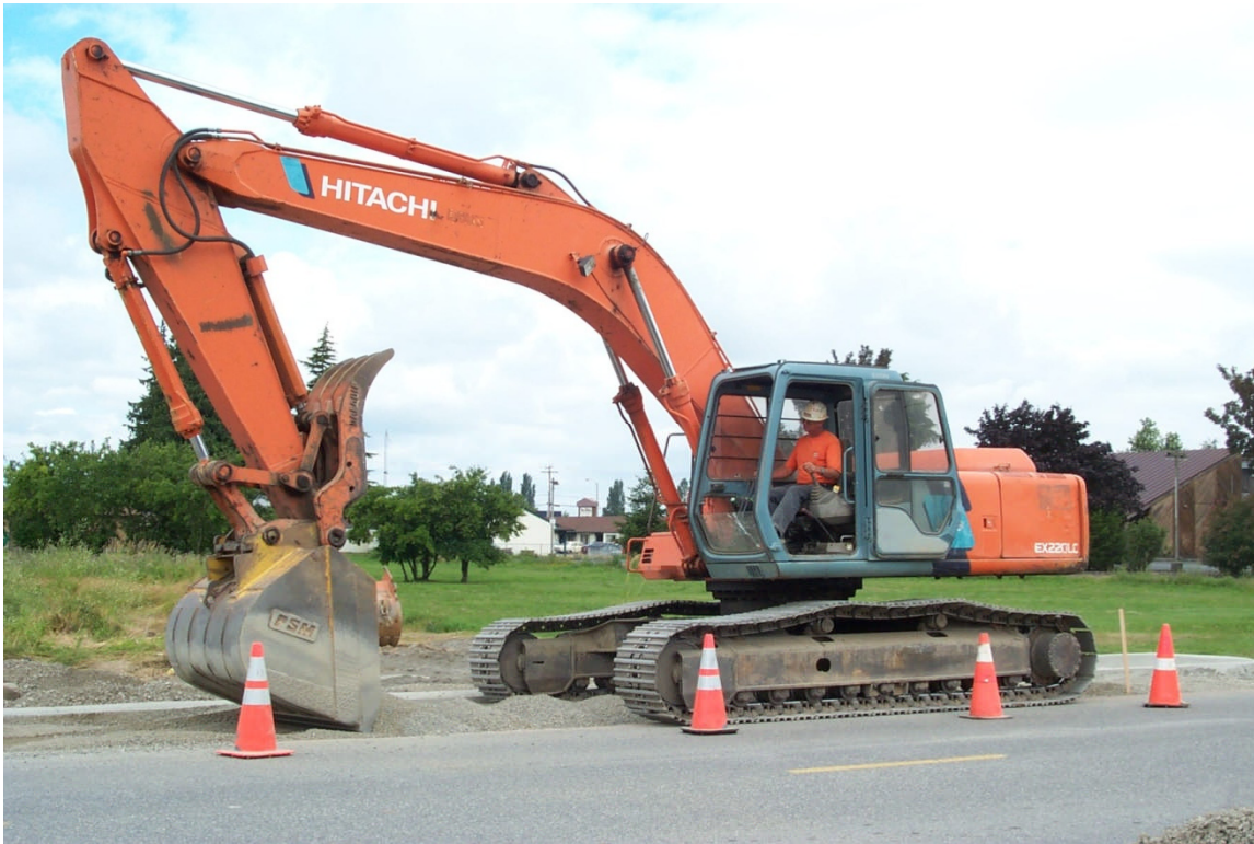
Road improvement project
